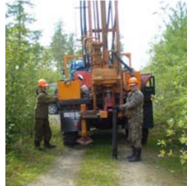
Drilling rig URB 2-A-2 based on an automobile URAL-4320
